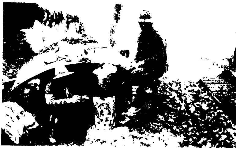
66. AUSTRALIANS IN IMPROVISED SHELTERS NEAR MONTAUBAN, WINTER OF 1916
